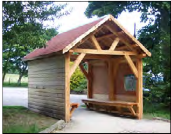
Shelter built by a Thistle Camp volunteer team
