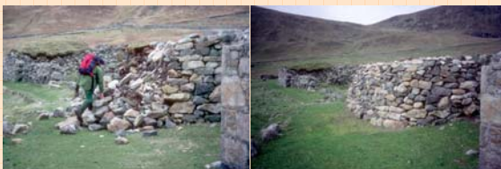
Blackhouse before and after restoration
