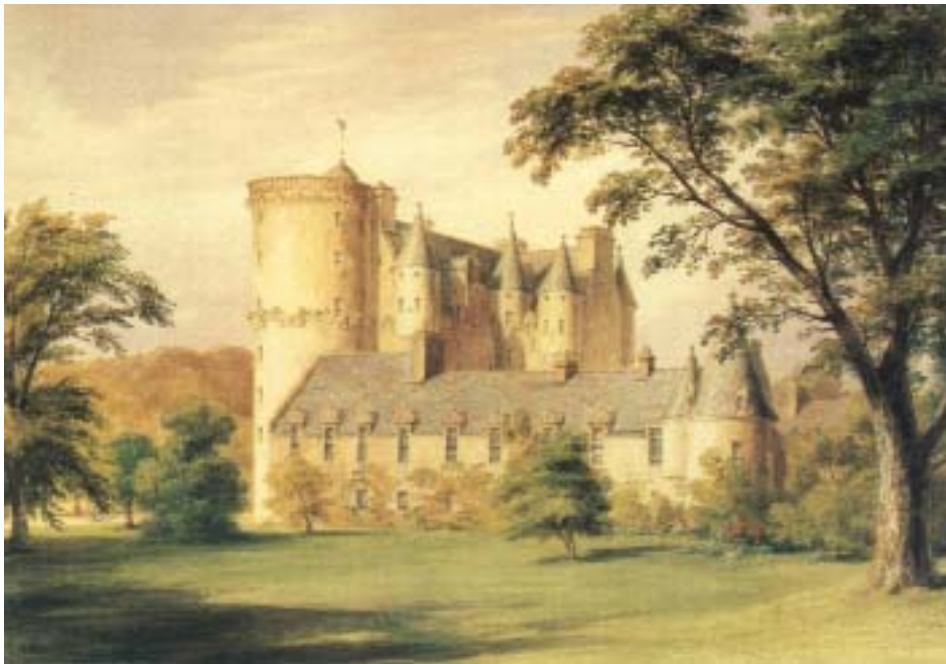
Completed around 1633-6, a first-floor gallery in this wing would have had a spectacular view of formal gardens occupying the lawn area in the foreground.
