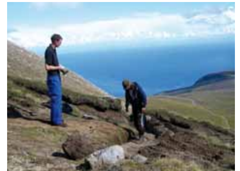
Laying stone at Coire Lan, Arran
