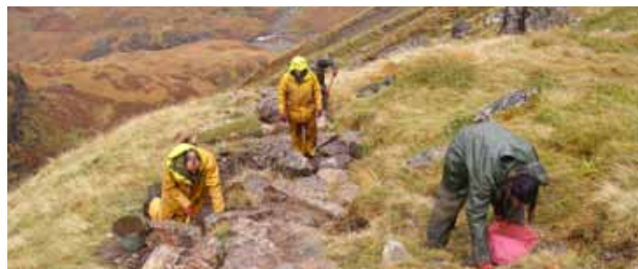
The MPMT carrying out landscaping repairs in Coire nan Lochan, Glencoe
